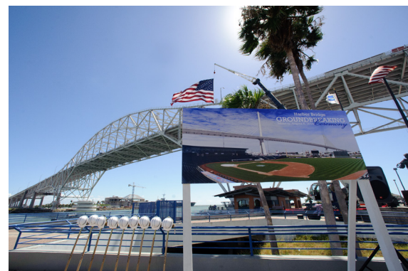
Groundbreaking for the US 181 Harbor Bridge Project
