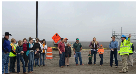
Engineer Chris Ursery explains the process of how the new bridge will be built at the January Sidewalk Talk.
