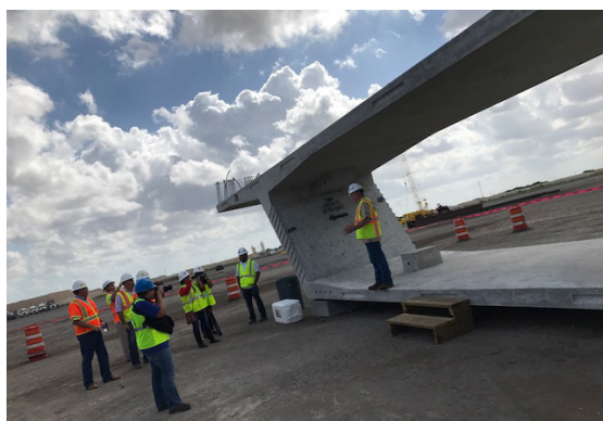
Darrell Chambers, FDLLC MOT Manager, talks to local media about the process of casting segments.
