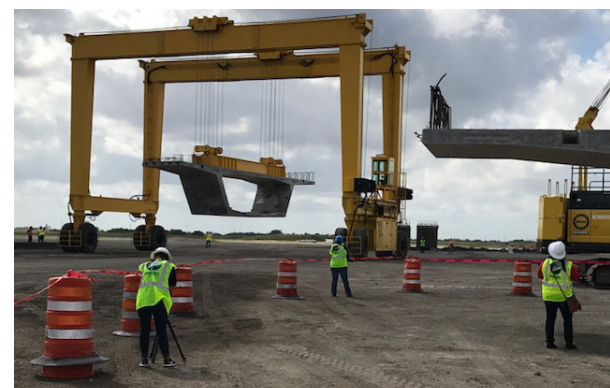
Local media capture movement of a 100-ton segment at the Pre Cast Yard in Robstown.
