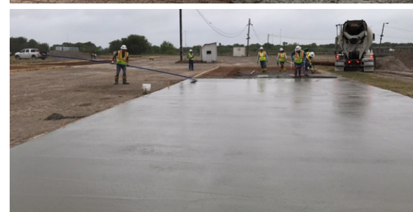
FDLLC employees pour concrete for one of several slabs at the Flato Road concrete batch plant.
