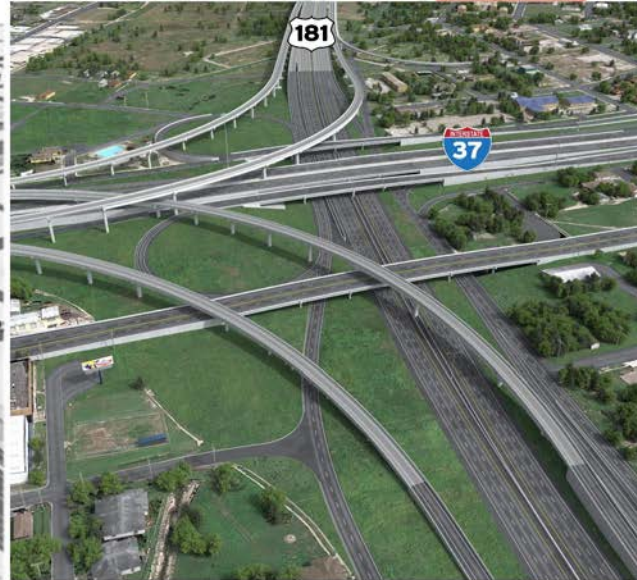
Enhanced Interchange Creating Multiple Free Flowing Connections
